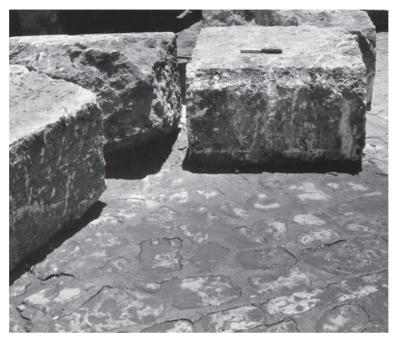
Fig. 4. Ashlar blocks with hammer dressed margins.
